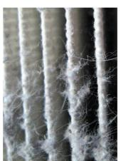
**Bio-growth and mold** coated coils and components can be a health hazard. They also insulate cooling fins and readily attract dirt and debris, taxing equipment and wasting energy. Indoor air quality is compromised as spores and bacteria are passed with supply air to living and working spaces.
