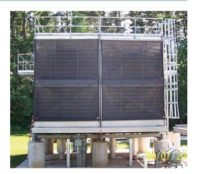
**So, what's the big upside of this?** Cottonwood Filter Screens increase the evaporative capacity of the Fill, reducing water temperature at the basin by 1 to 2 degrees Fahrenheit beyond its original design temperature. This translates into a significant reduction/elimination in downtime, lost productivity and energy savings.
