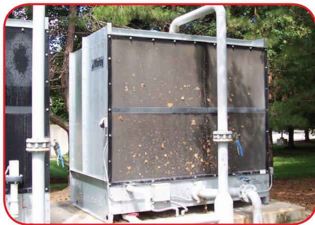
Keep bugs and debris out of cooling tower Intakes.
