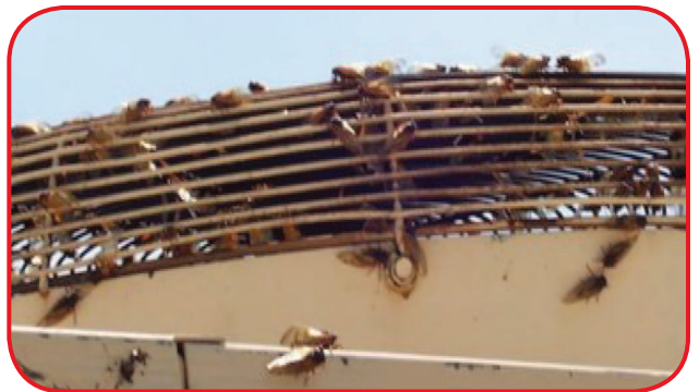
Cicadas entering motor vents cause fan motor damage.
