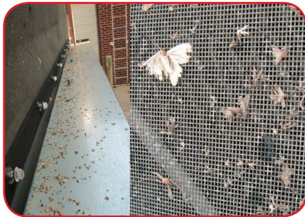
Cottonwood filter screens effectively stop small insects.
